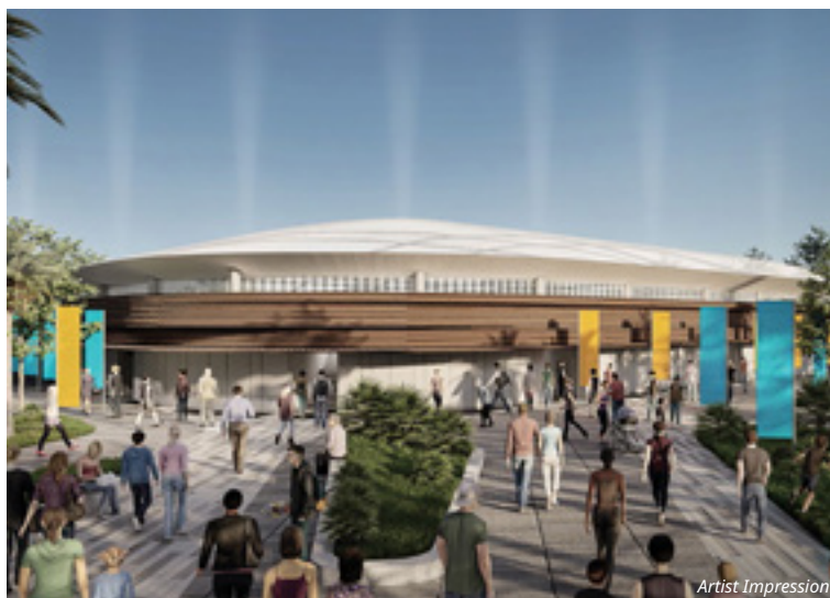
Queensland Tennis Centre, Tennyson
